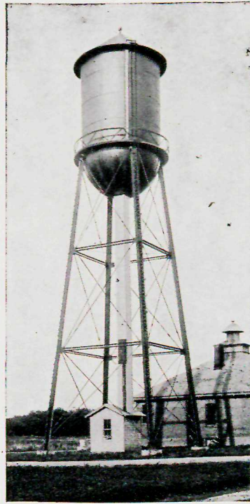
WATER TOWER, HAZEN, N. D.
